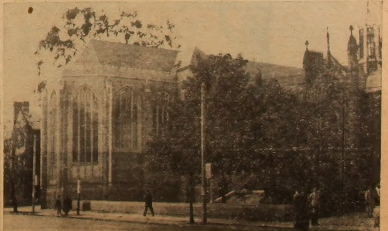
Trinity's new chapel and stone wall are shown here. The chapel is now structurally complete but will not be officially open until the beginning of November. —VSP by John Ellis
